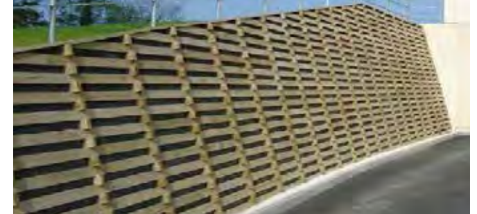
Cribblock retaining wall
