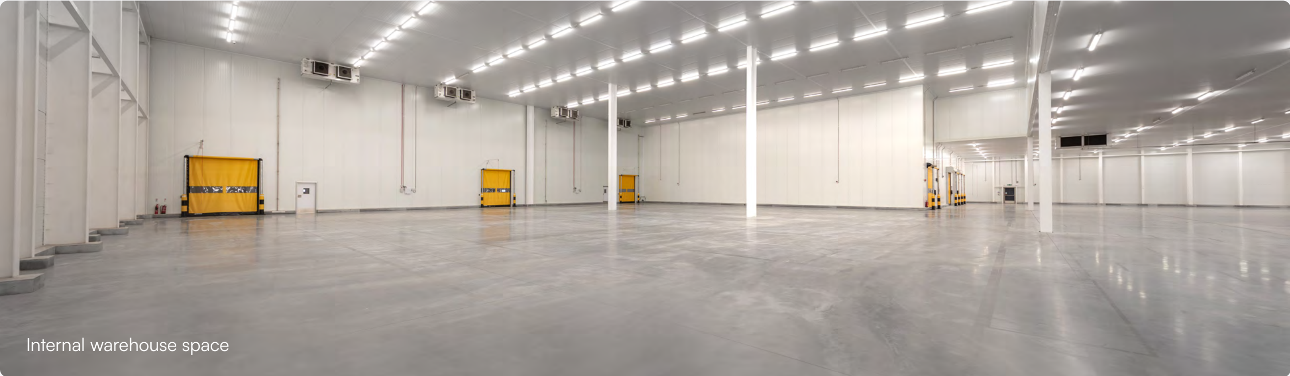
Internal warehouse space
