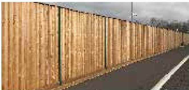
Typical Acoustic Barrier
