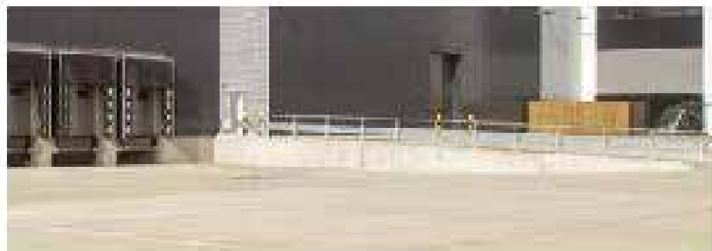
Acoustic retaining wall with backlit lighting
