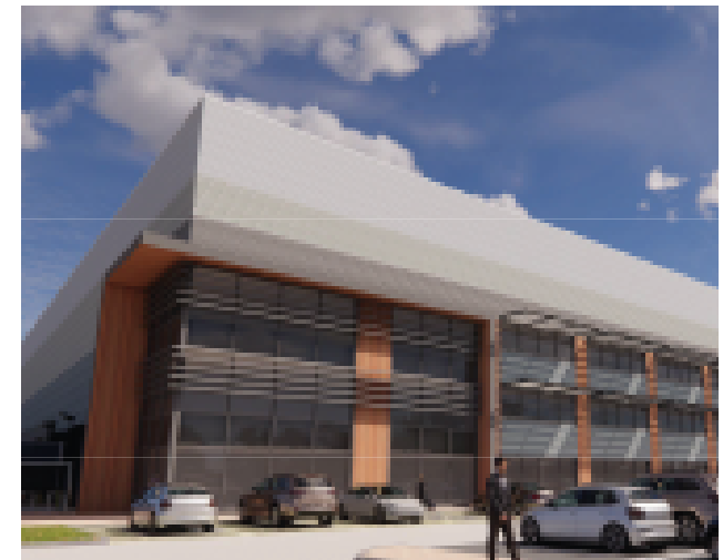
Solar shading to southern elevations
