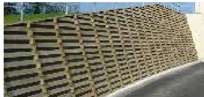
Acoustic retaining wall
