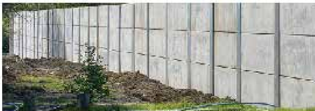
Acoustic retaining wall with noise barrier, suitable for public areas
