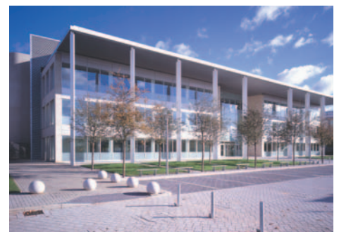
200 Bath Road, Slough.
