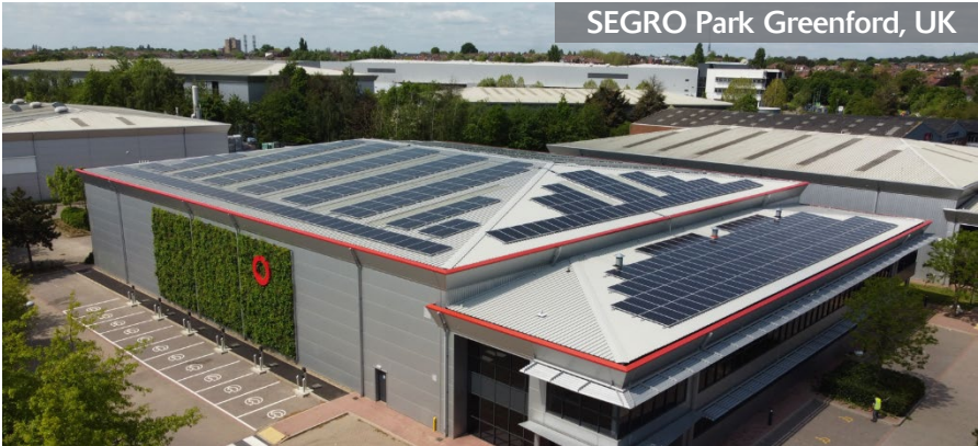
Highly sustainable refurbishments
