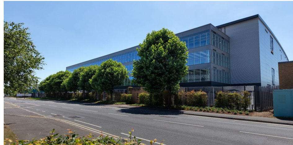
Iron Mountain, Slough Trading Estate
